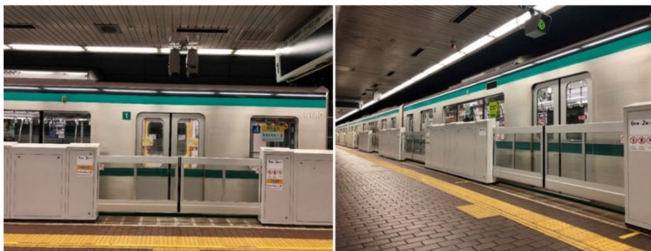
Figure 2 Installation of platform doors on No.1 platform of Shin-Nagata Station
