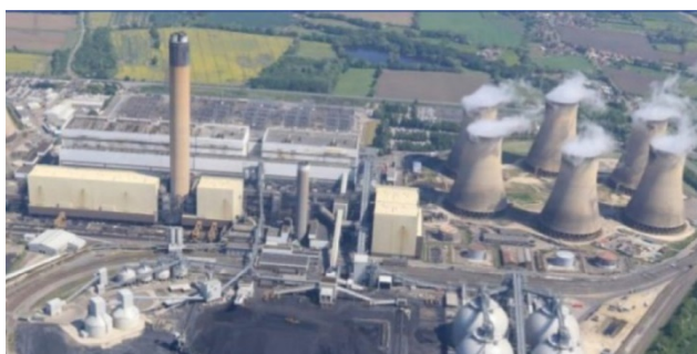
Figure 5 DRAX's biomass power generation plant (4)
