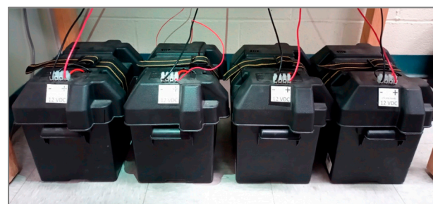
Figure 9. Battery bank.
