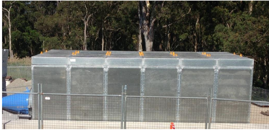
Figure 4. Stage 1 bottom ash-based enclosure outside the detonation tube in silencer area.
