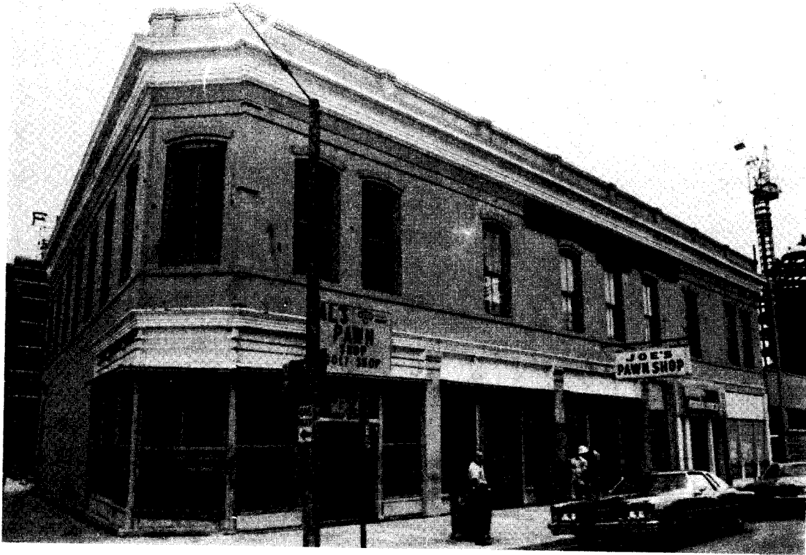
FIGURE 5-18 SOUTH FACADE OF THE A.R. COGSWELL BUILDING
