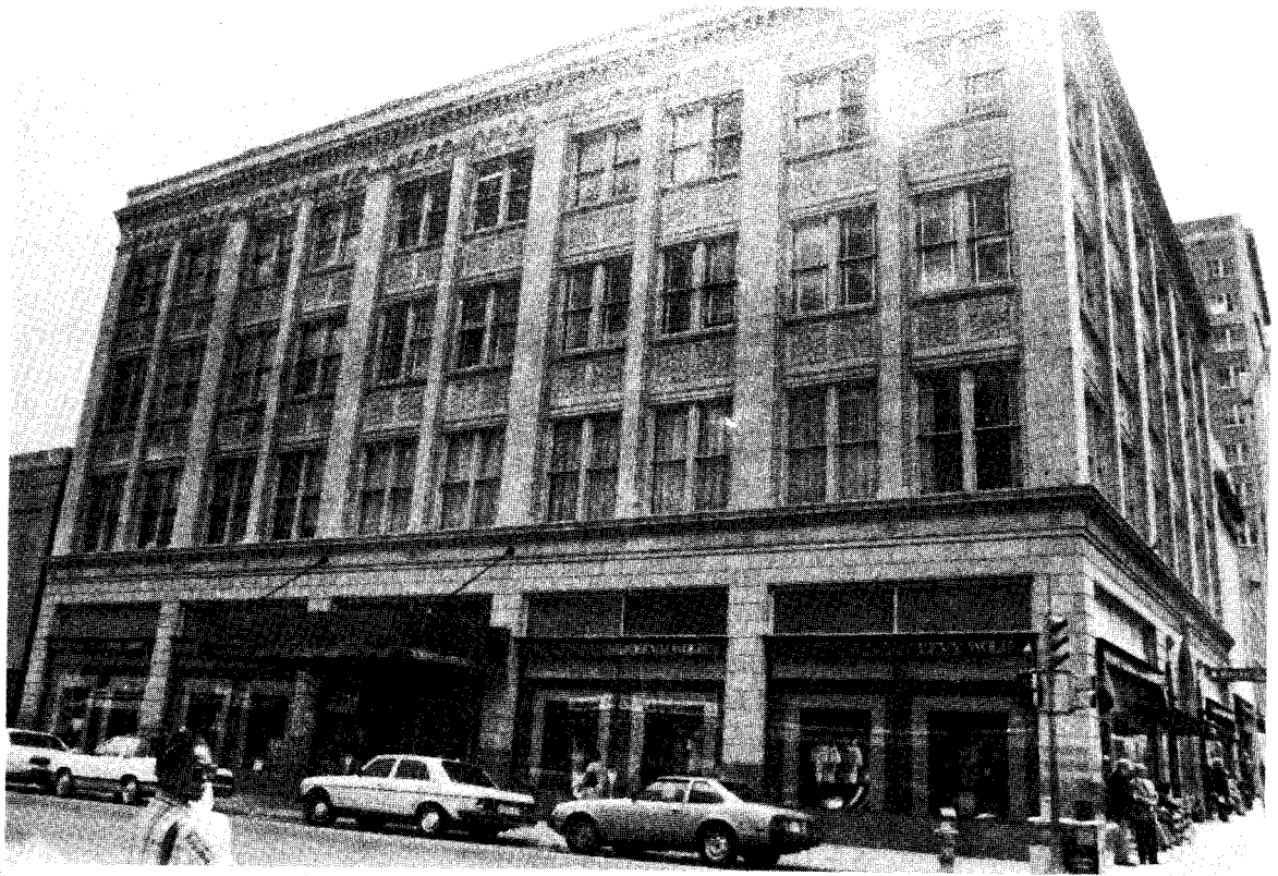
FIGURE 5-16 SIDE ENTRANCE ON THE WEST FACADE OF THE LEVY-WOLF BUILDING
