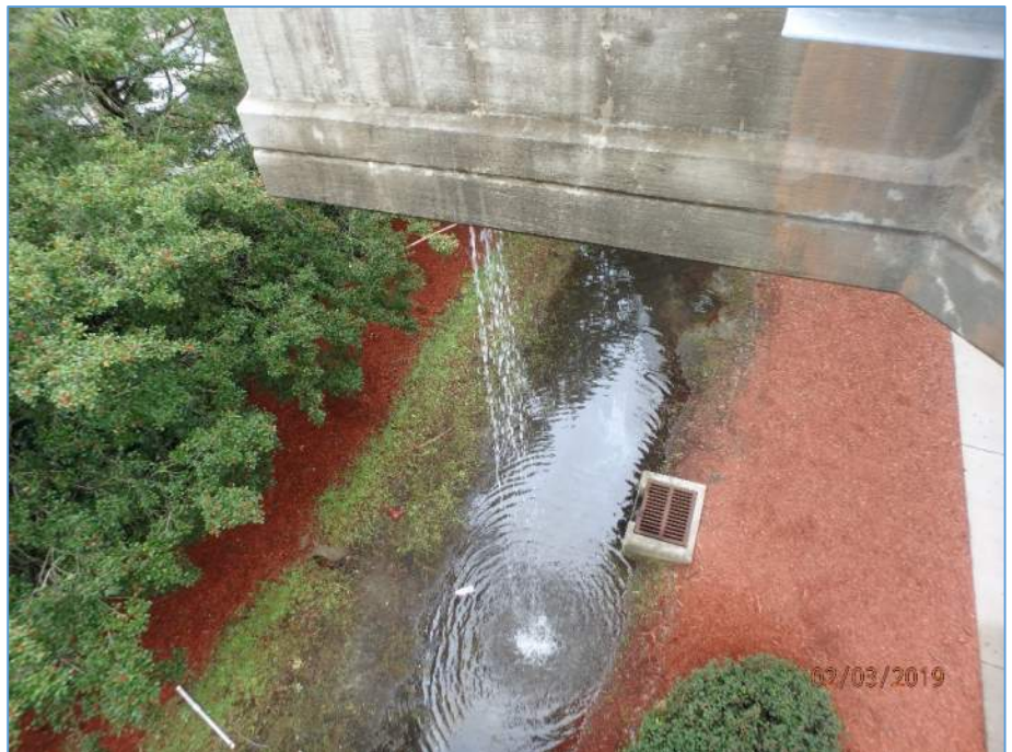
Span 205L: Water Draining from Deck after Debris Removal
