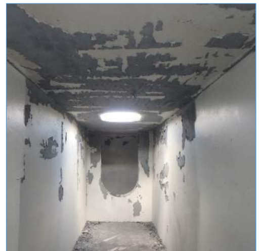
Pier 10 Cross Girder
