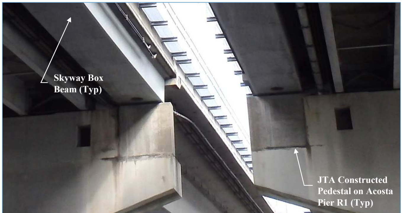
Acosta Bridge Pier R1 Supporting Guideway Superstructure (Photo from the 2017 Inspection)
