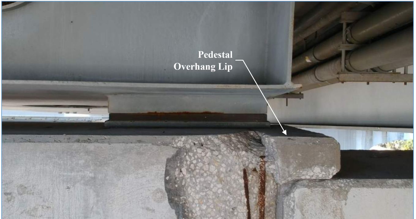
Close-up of Acosta Bridge Pier R1 Left, Front Face
