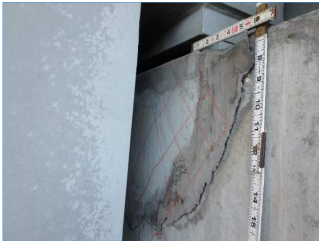
Pier 258L: Large Delamination Below the Right Bearing, Rear Face
