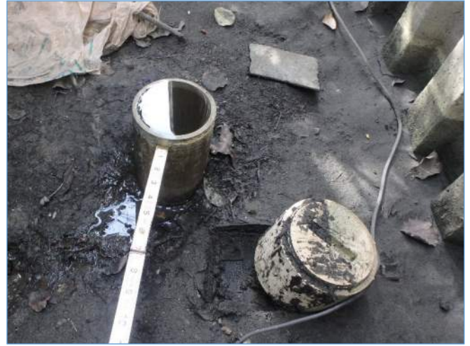
Span 253R: Riser Pipe Filled with Water
