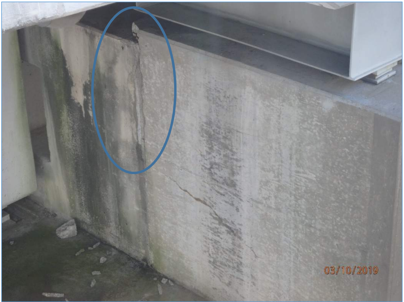
Acosta Bridge Pier R1 Right, Front Face
