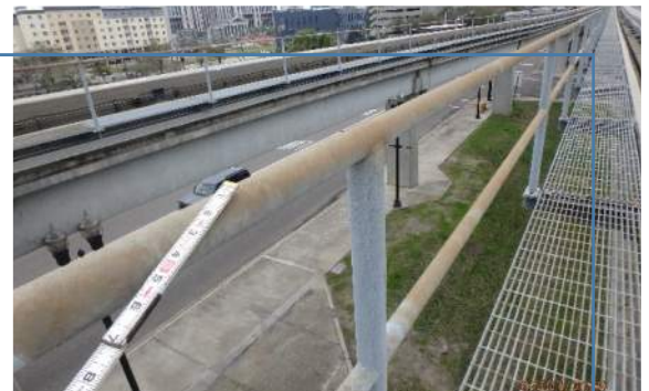
Handrails and Posts
