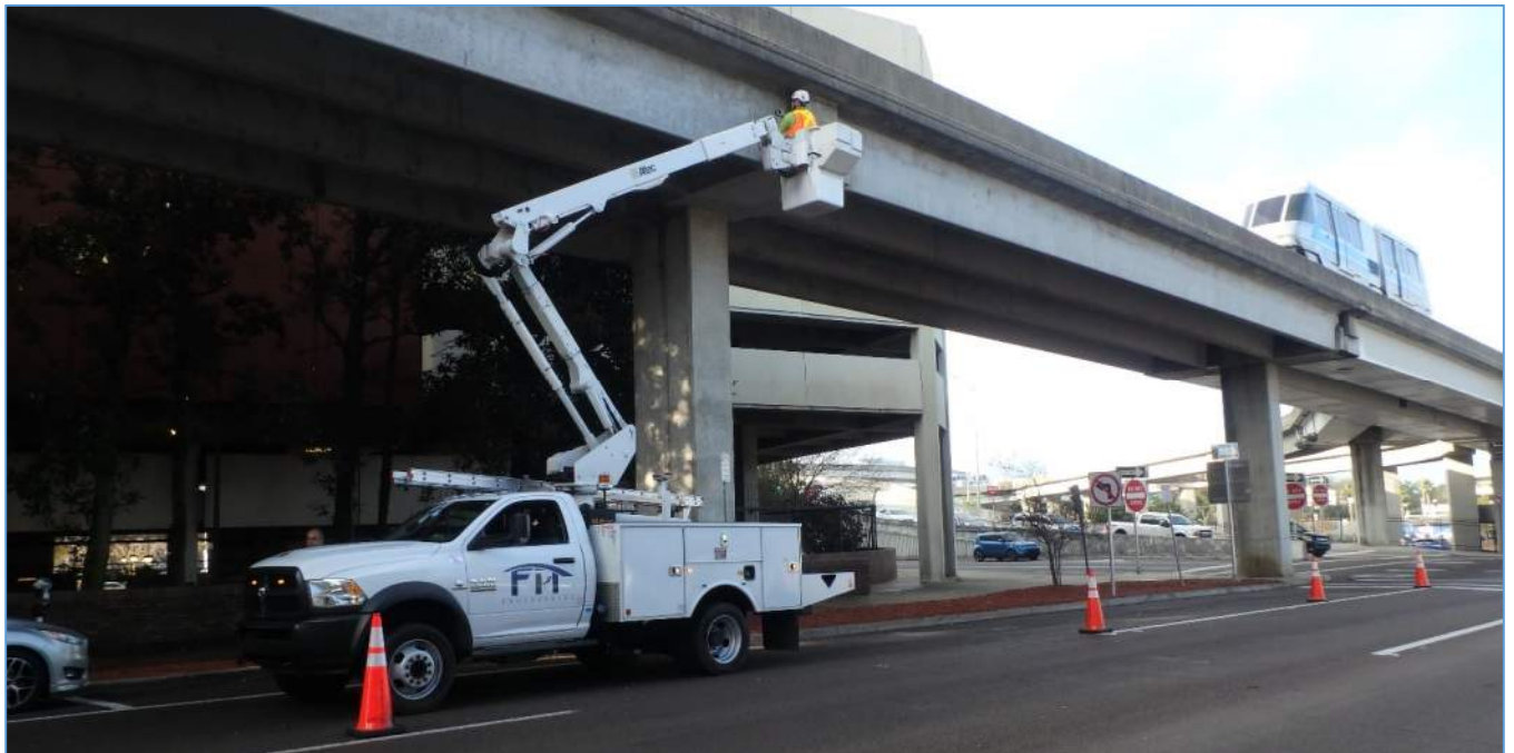
Bucket Truck Use to Inspected Concrete Beams along Bay Street
