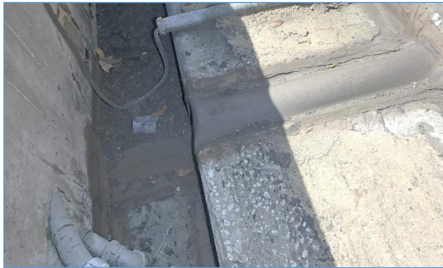
Pier 62L: Joint Covered With Neoprene Seal (Photo from 2017)
