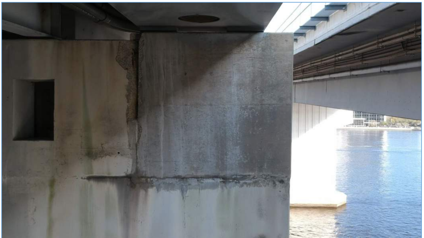
Acosta Bridge Pier R1 Left, Rear Face
