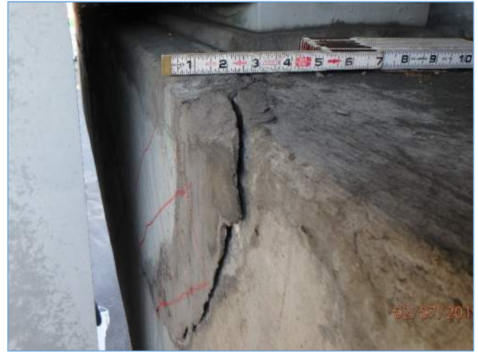
Pier 258L: Large Delamination Below the Right Bearing, Rear Face
