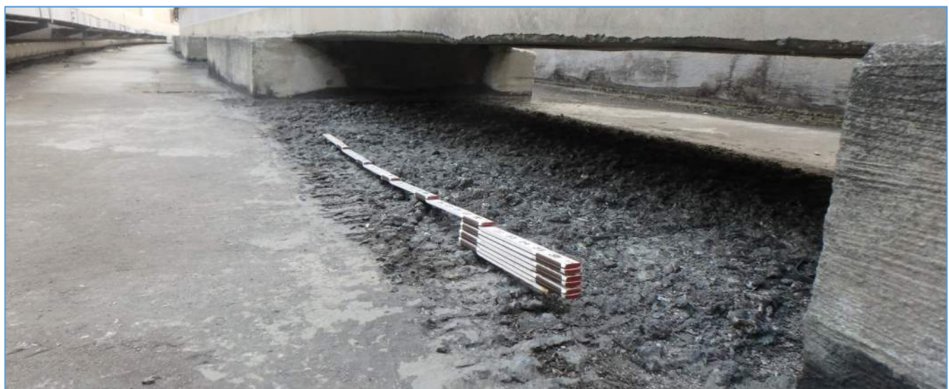
Typical Roughened Deck Top in the South Line
