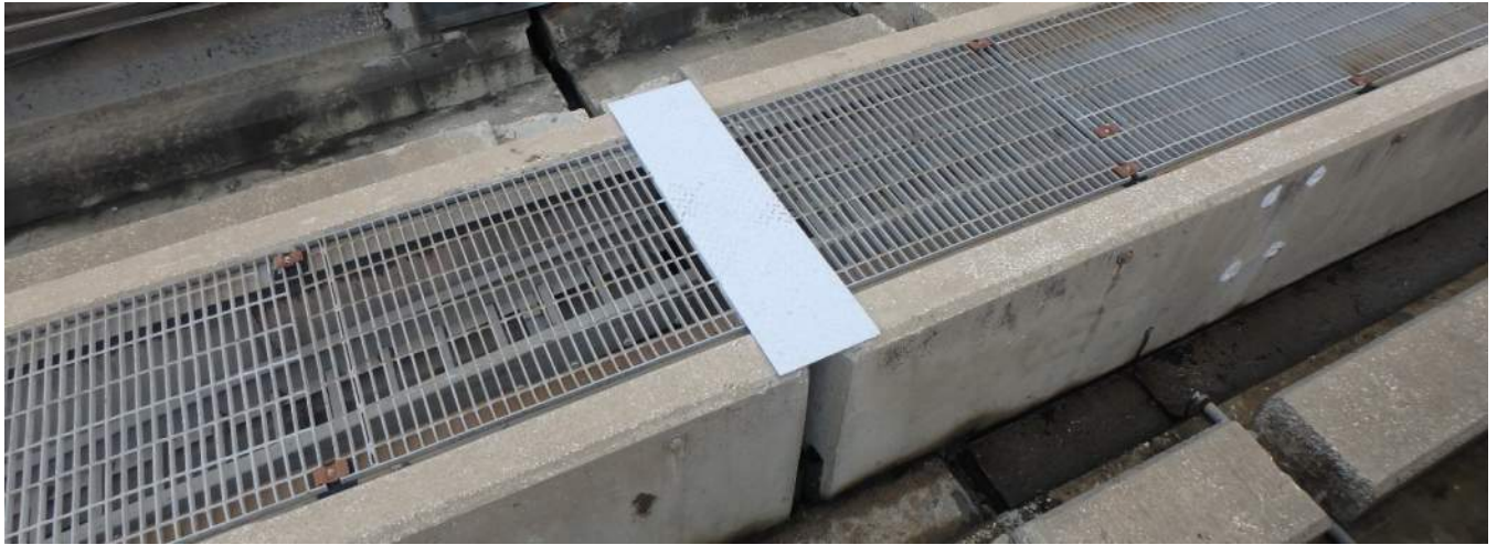
Coated Emergency Walkway Grating Expansion Cover Plate at Pier 32
