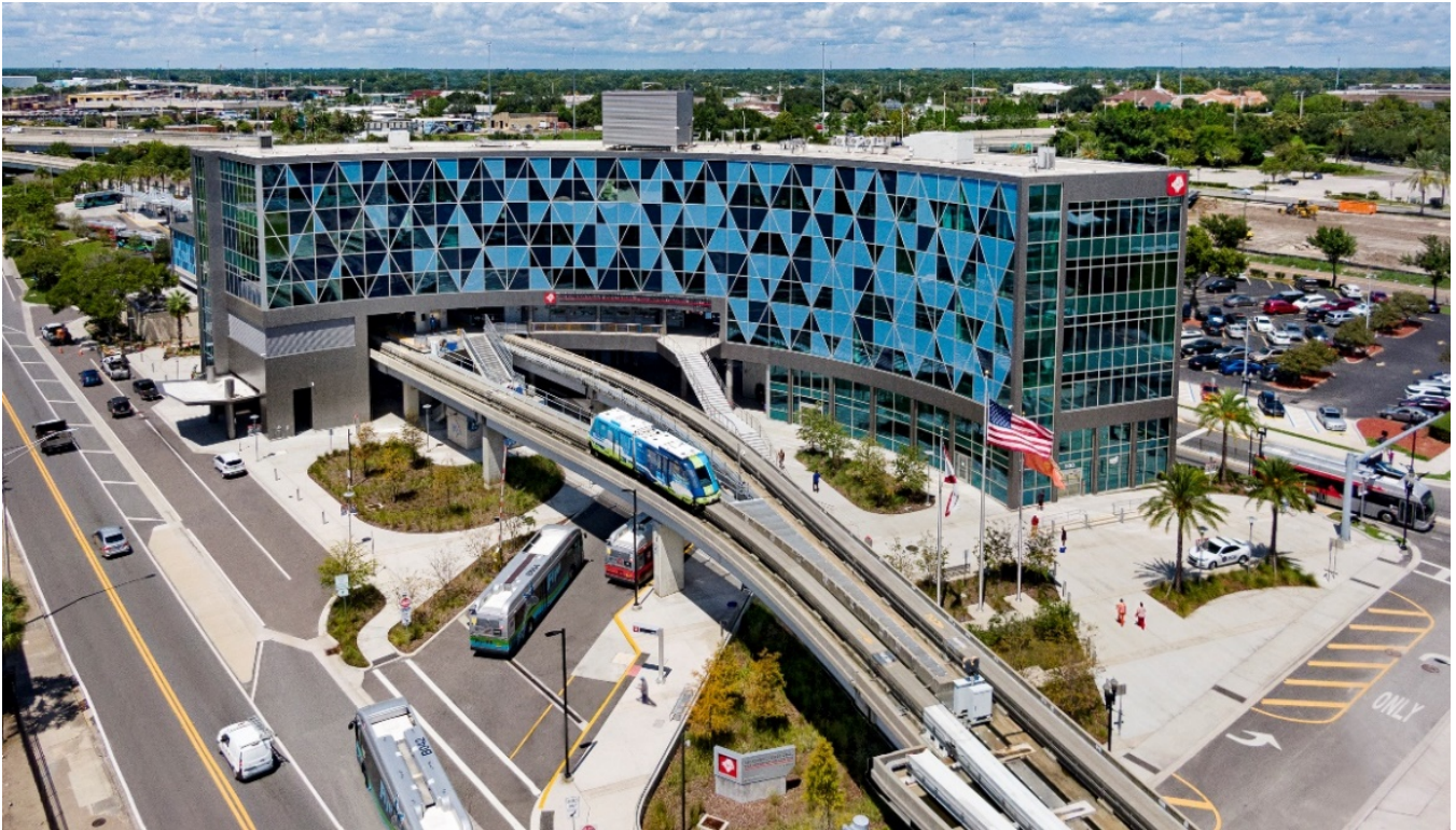
Figure 7. The Jacksonville Regional Transportation Center
