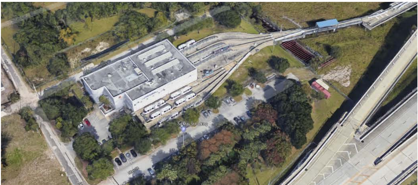
Figure 4. The JTA's Skyway Operations and Maintenance Center
