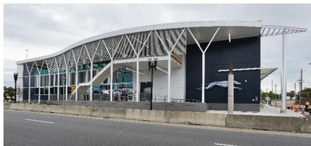
Intercity Bus Terminal, Opened January 2018
