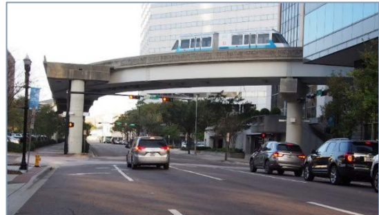
Skyway Infrastructure at Bay and Hogan
