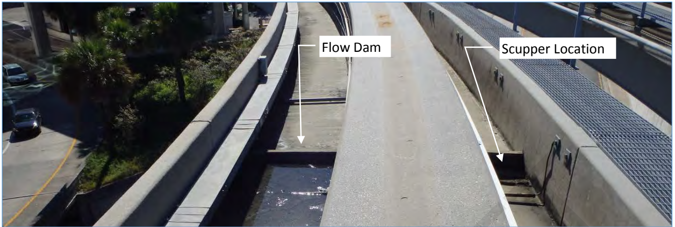
Pier 242 RT. Guideway, Looking Back
