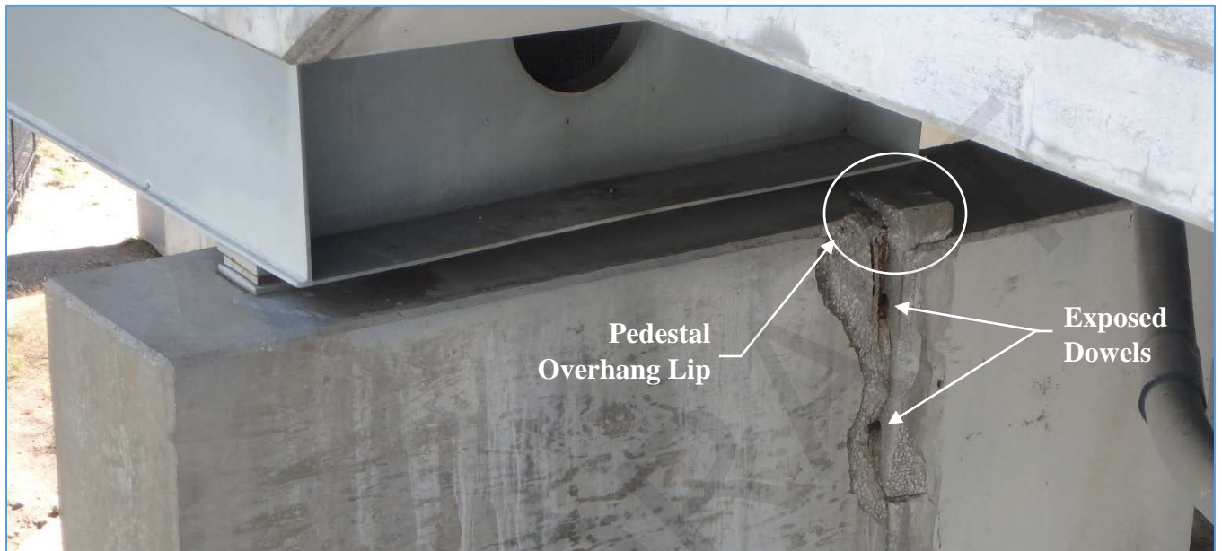
Acosta Bridge Pier R-1 Left, Rear Face
