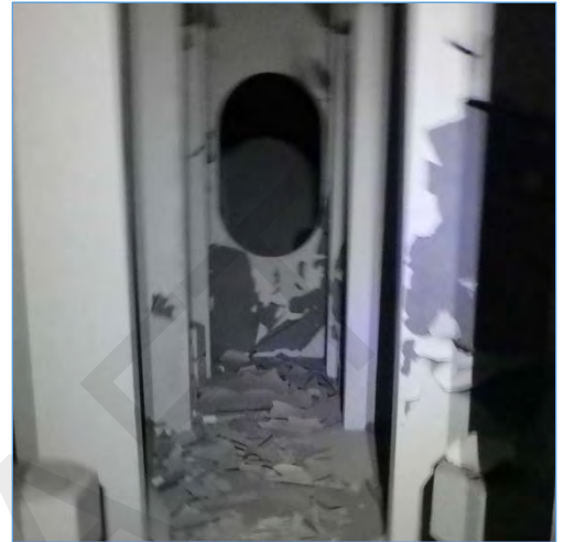
Pier 11 Cross Girder
