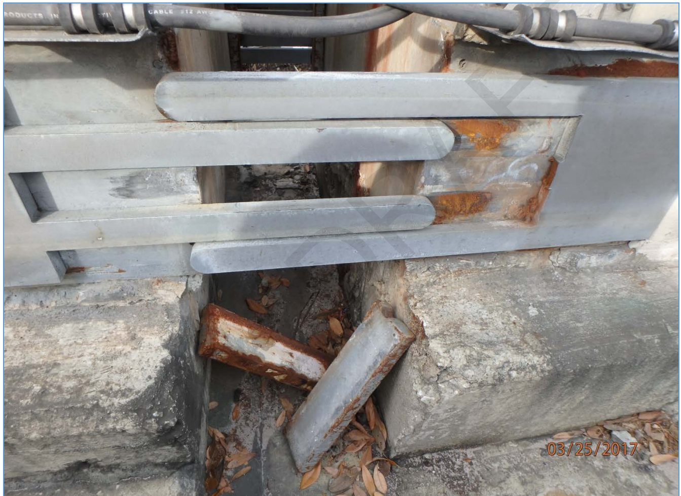
Pier R-6L, Guidebeam Expansion Joint, Right Side
