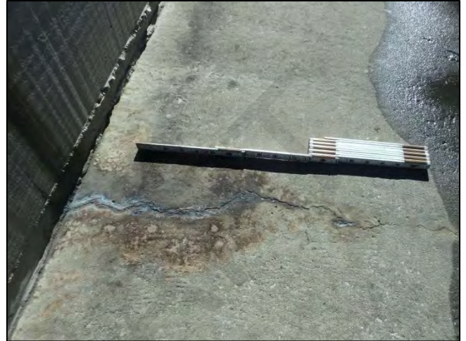
Span 241: Transverse Cracking on Deck Top Surface
