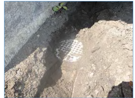
Buried Drain Cap at Pier 409R
