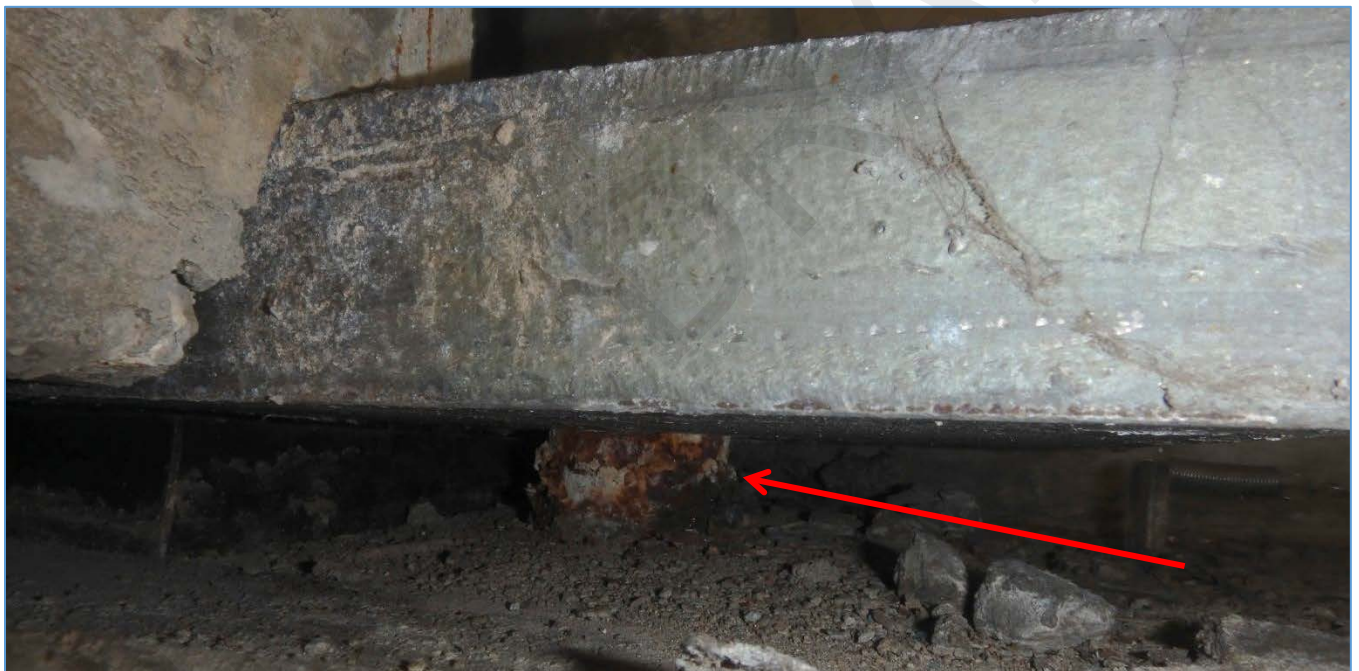
Span 239L at Pier 240L: Surface Corrosion on Bearing Plate Anchor Bolt
