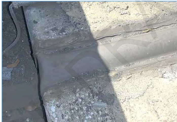
Pier 62L: Joint Covered With Neoprene Seal
