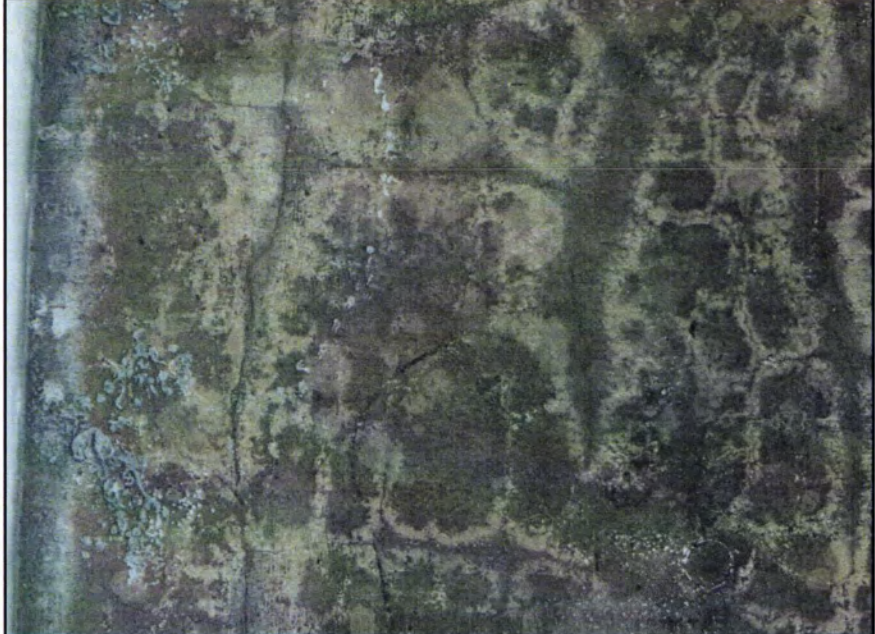
PHOTO 23 – ELEMENT 220 TYPICAL VIEW OF THE INSIGNIFICANT SIZE LONGITUDINAL, TRANSVERSE AND DIAGONAL CRACKS IN THE TOP OF FOOTINGS
