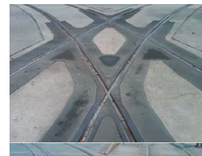
Figure 4-20: Embedded Track Diamond
