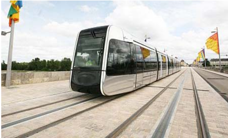
Figure 4-4: Alstom Citadis guide rails and APS embedded power rail, Tours, France (Image: Alstom, www.raillynews.com )
