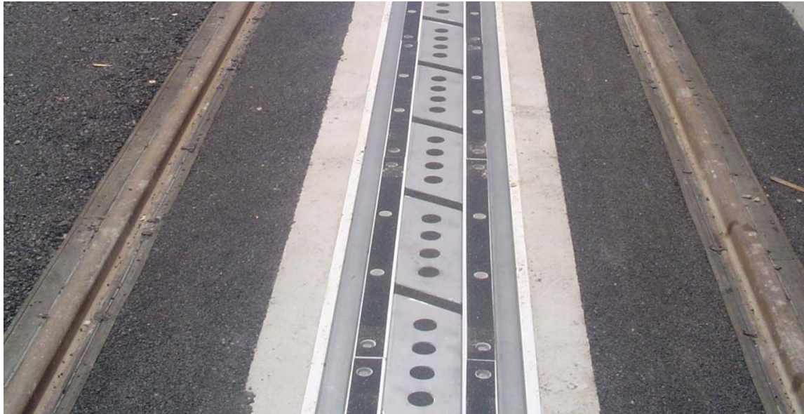
Figure 4-26: Embedded Power Rail (Stream by Ansaldo-Breda)
