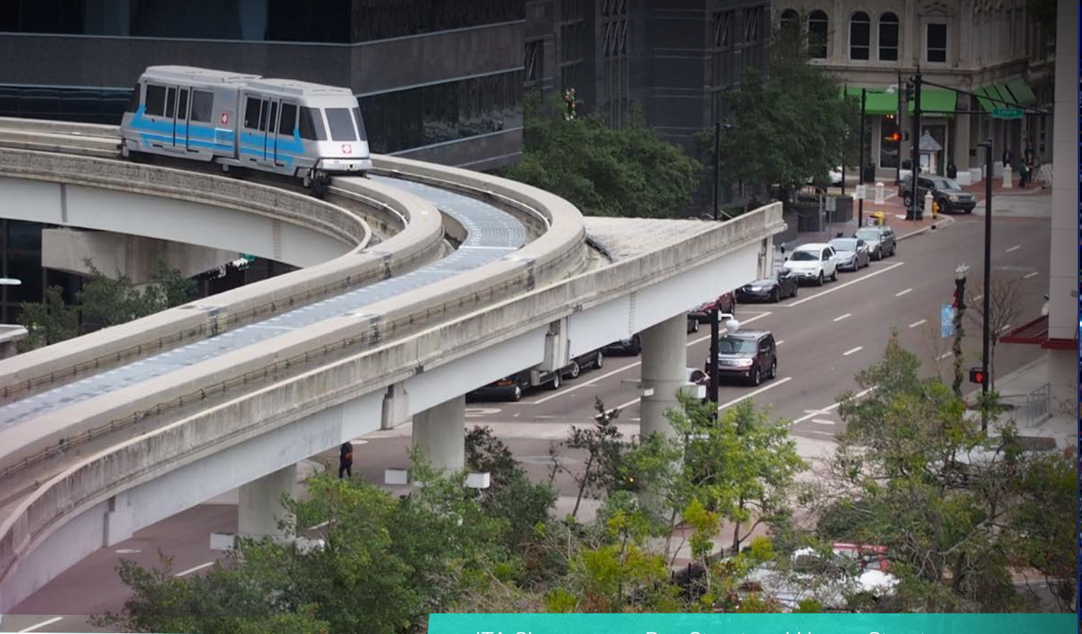
JTA Skyway over Bay Street and Hogan Street
