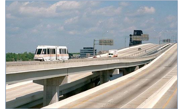
Elevated Skyway – Acosta Bridge
