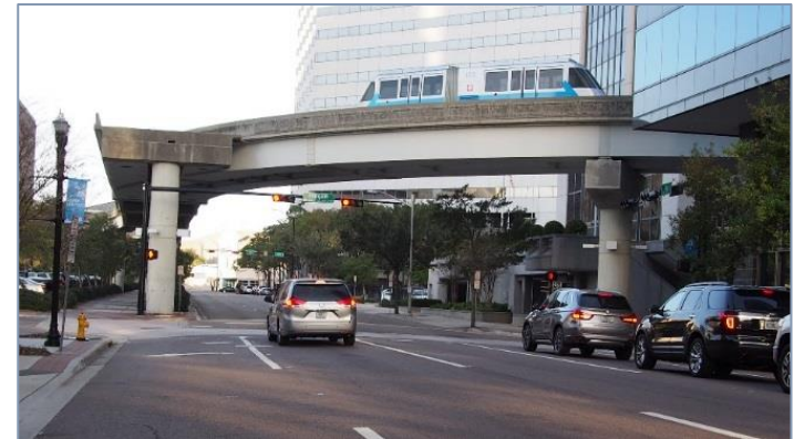
Skyway Infrastructure at Bay and Hogan
