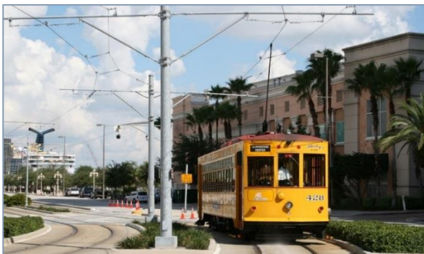
Overhead Catenary Example – Tampa TECO
