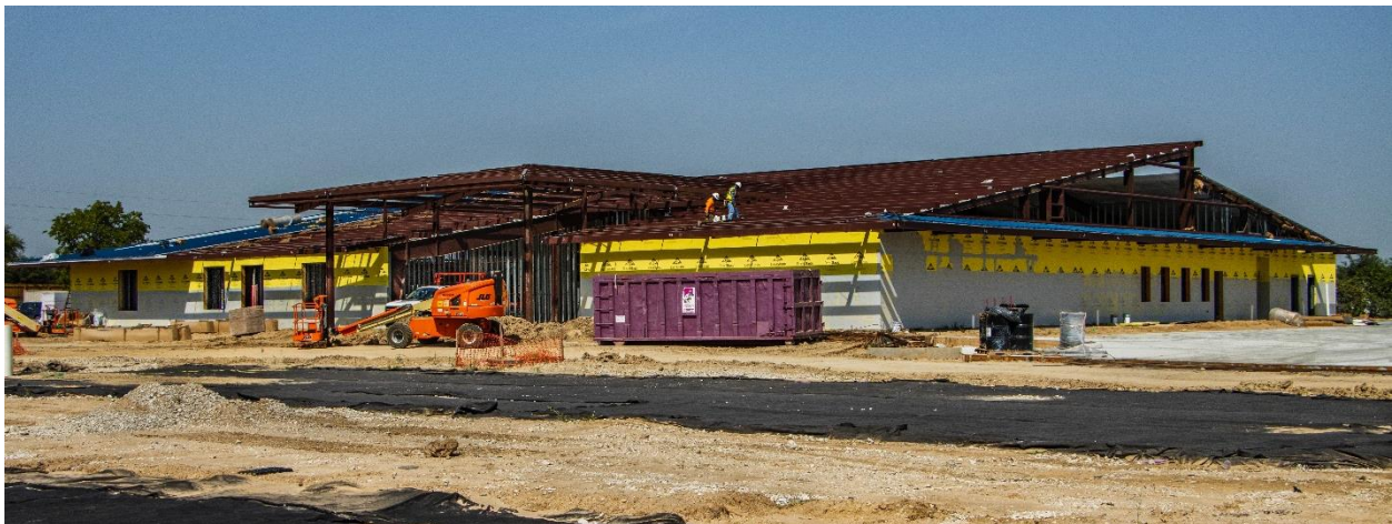
Clay Road Community Center construction about 50 percent complete.
