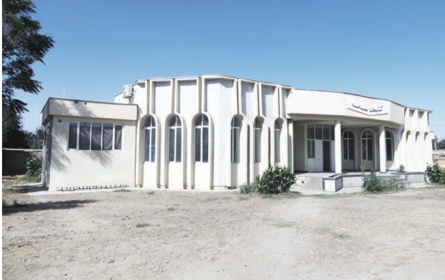
The Kunduz library constructed with funds from the Good Performers Initiative, Kunduz Province. (SIGAR photo)
