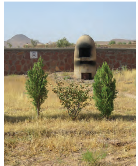
SIGAR's site inspections of USAID-supported health facilities in Herat Province revealed some concerns, including open-air kilns used for disposing medical waste, raising the risk of exposing patients and nearby children to contaminated waste. (SIGAR photo)
