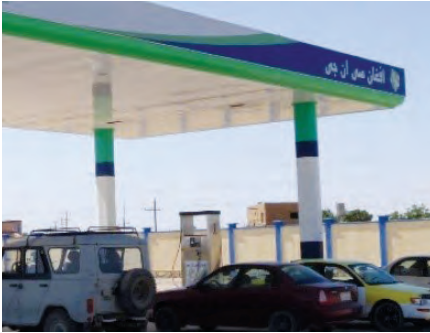
TFBSO's Downstream Gas Utilization project, which constructed this compressed-natural-gas filling station, was the subject of a SIGAR special project review this quarter. (Central Asia Development Group photo)
