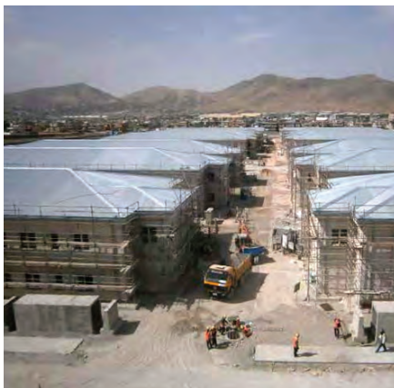
The MOI headquarters administration buildings are located in Kabul. (CSTC-A photo)
