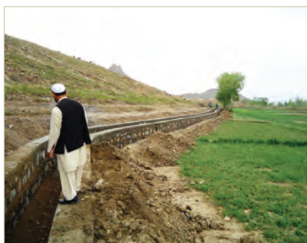
A SIK-East canal project in Paktiya Province in May 2015. (USAID photo)
