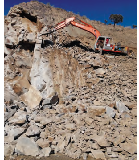
Construction of the Gardez-Khowst road is ongoing. (USAID photo)
