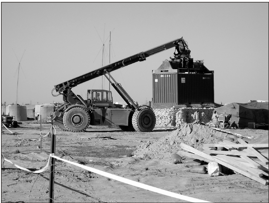
Heavy demand on support equipment.
