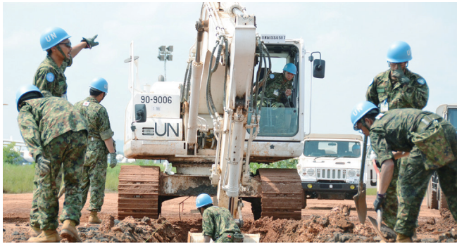
GSDF personnel conducting ditch construction in South Sudan
