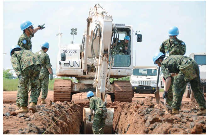
SDF personnel conducting gutter maintenance in South Sudan
