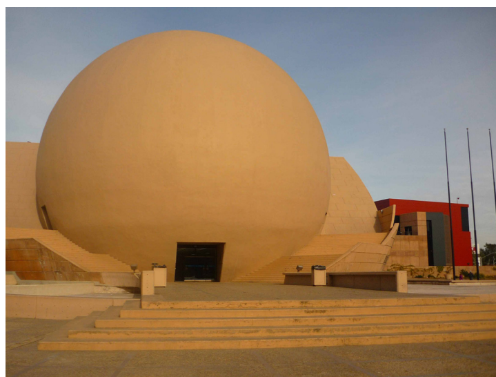
Exterior view of the IMAX dome in Tijuana, Baja California, Mexico.
