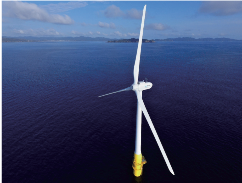
Photo 2 Goto City's Sakiyama 2 MW floating offshore wind power plant (Photo by Toda Corporation)
