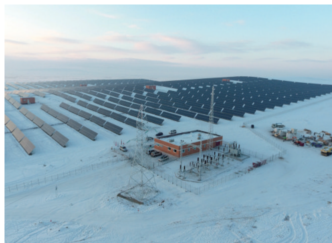
Photo 2 10MW Solar Power Project in Darkhan City, Mongolia
