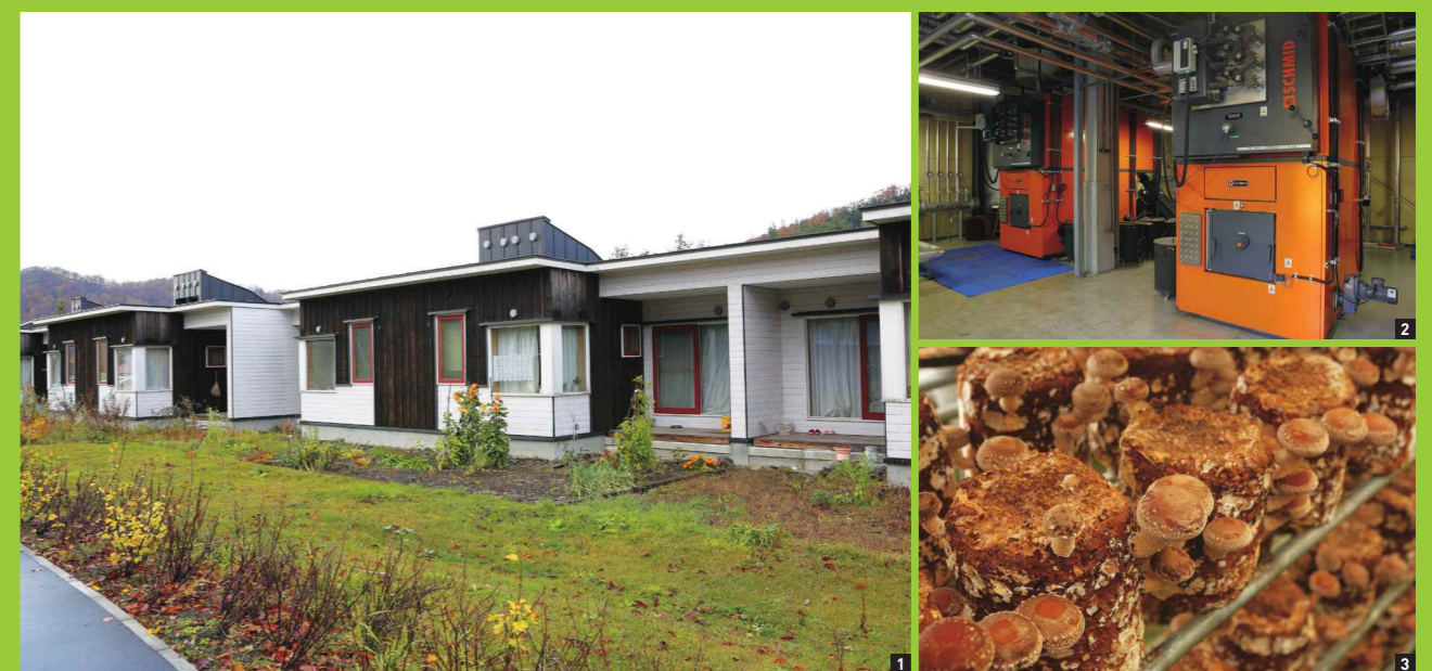
1 Ichinohashi Bio Village residential buildings. They are connected by shared indoor corridors, making it easy to start up a conversation with neighbors. 2 The biomass boilers installed in Ichinohashi Bio Village. The two 550kW boilers provide heating and hot water for the community. 3 In this plastic greenhouse that uses the heat from the boiler, shiitake mushrooms are cultivated in beds that use sawdust from the trees, creating employment for local residents.
