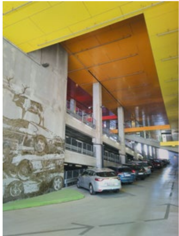
Fig. 7 Ørestad: wall relief in the parking garage of the MTN housing project, BIG. (Source: Björn Hekmati)
