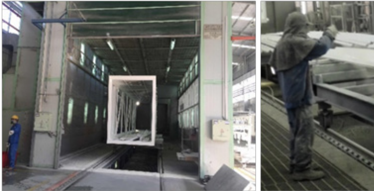
Figure 1. The current painting process for the boarding bridge.
