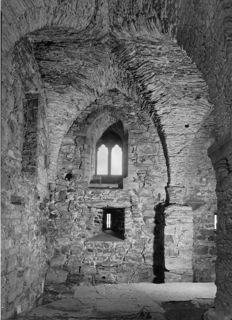
Fig. 7.7: The royal palatium at Holmen. King Håkon's hall, the two lower stores during restoration in the 1950s. The vaults, built after the fire in 1266, are constructed with thin flagstone. Photo: G. Fischer. Source: The Directorate for Cultural Heritage.
