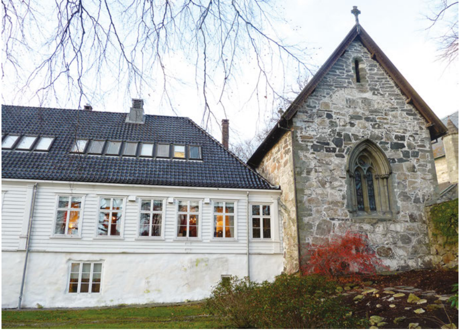
Fig. 7.33: Stavanger. The bishop's palace. The wing's basement in stone (now plastered) related to the two-stored bishop's chapel with the chapel itself in the first floor, viewed from the east. Photo: A. T. Hommedal.
