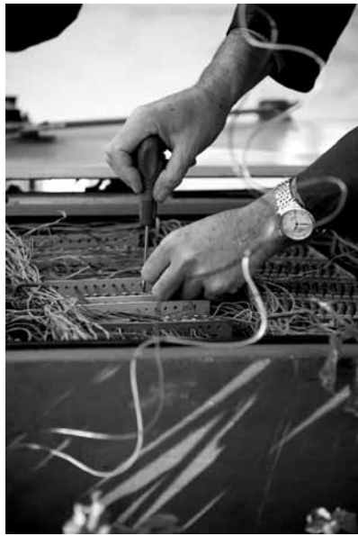
Fault management by OTE technicians
