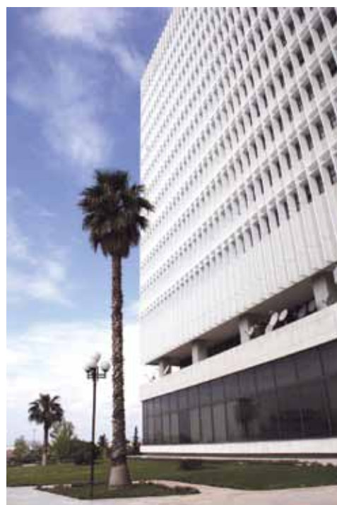
OTE headquarters building
