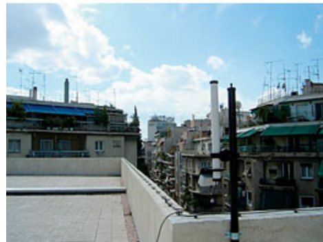
24-hour electromagnetic radiation monitoring station
