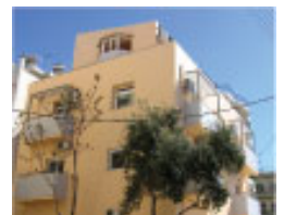
The "IRIS" Adolescent Hostel of the "Association for the Psychosocial Health of Children and Adolescence", the construction of which COSMOTE contributed to for many years
