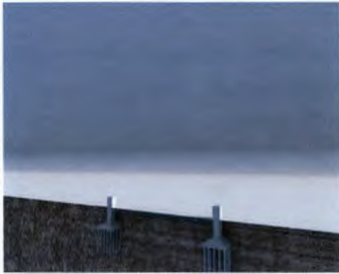
Step 1: Foundation and piling of "Dubai Frame". Erection of tower with climbing formwork.
