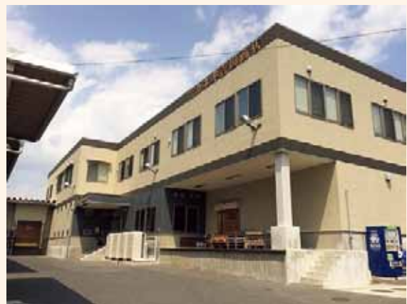
The company's rebuilt Number 2 plant
