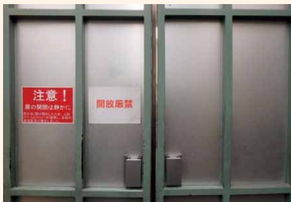
Aluminum doors that are easily opened and closed in the event of emergency
