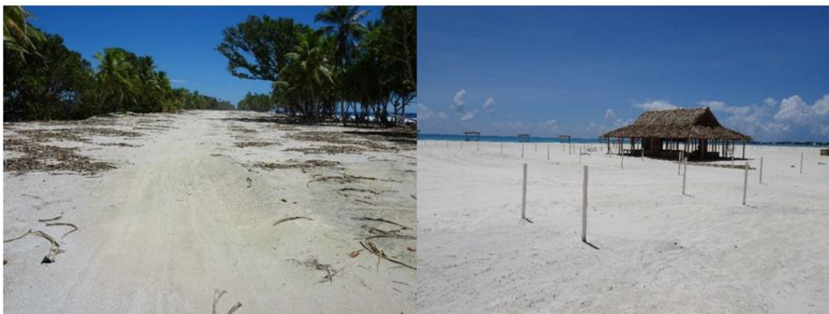
Figure 6: Former borrow pits north of the garbage dump reclaimed in 2014 and infilled with lagoon sediment dredged from Funafuti Lagoon (left); and the extensive reclaimed area on the lagoon side of the Tuvalu Government Building and Vaiaku Lagi Hotel, which was
