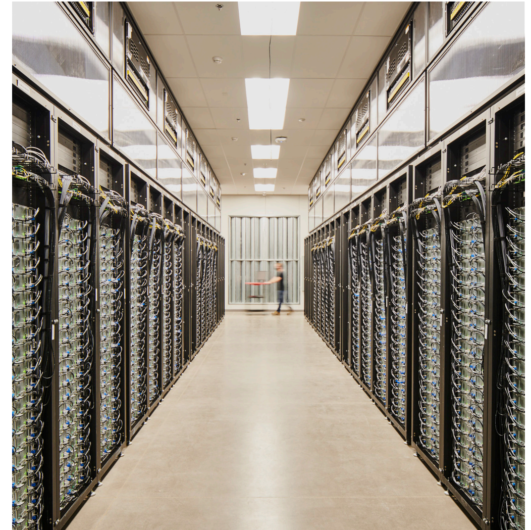
Apple’s Reno data centre, which opened in 2012, takes advantage of the mild climate by cooling its servers with outside air whenever possible.
