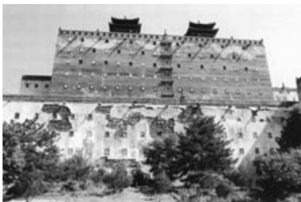
The Red Terrace of Putuozechengzhimiao before renovation, Chengde Mountain Resort, China
