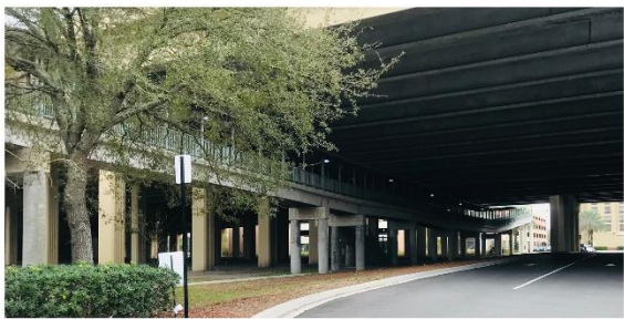
Footbridge under I-95 to Kings Avenue Parking Garage
