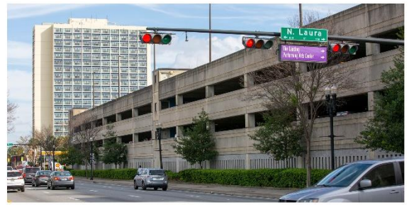
N Hogan Street Parking Garage
