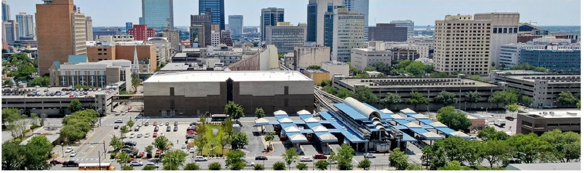
Aerial View of Rosa Parks Station
