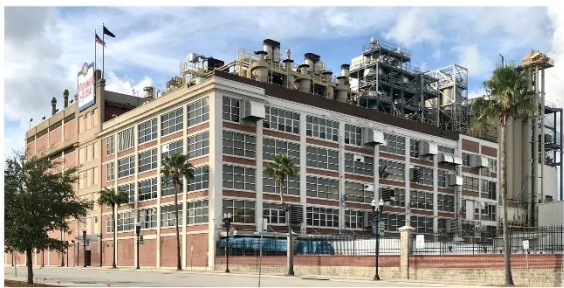
Maxwell House Manufacturing, Credit: WSP
