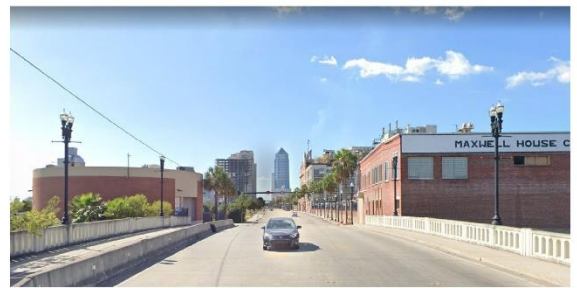
Hogan Creek Bridge, Credit: Google Streetview
