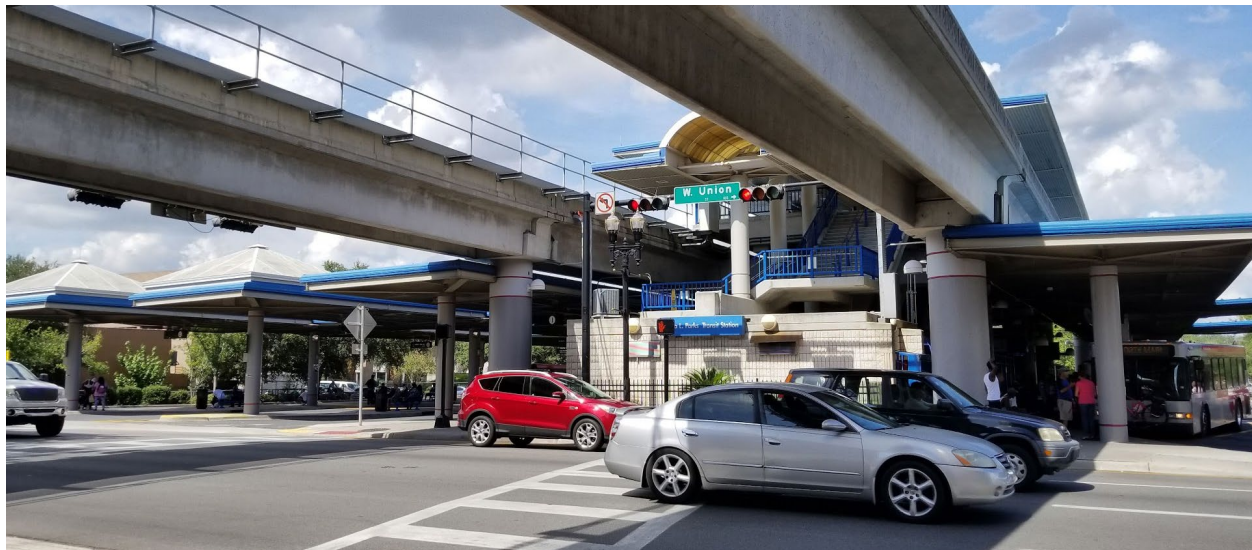
From an operational analysis, elevated extensions provide high reliability, short trips, and lower number of vehicles. Pictured above, elevated guideway over Union Street leading to Rosa Parks Transit Station.
