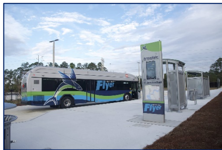
Curbside Station at First Coast Flyer
