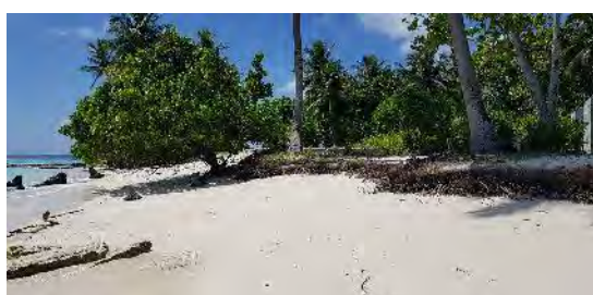
Figure 38.11: Eastern side - heavy erosion
