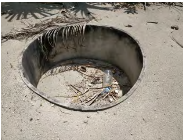
Figure 3.5: A few dug wells were observed throughout the island
