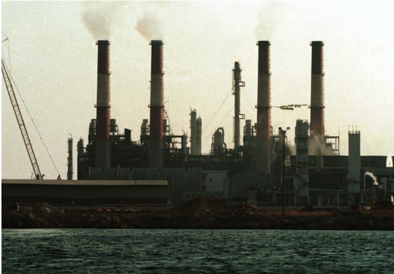
Fig. 4.5.5. A polyvinyl chloride production plant in Turkey. Occupational exposure to specific carcinogens such as vinyl chloride can be readily controlled through regulation of relevant concentrations in the workplace; control of occupational exposure to non-specific waste products, or their impact on the wider community, is more difficult to address.
