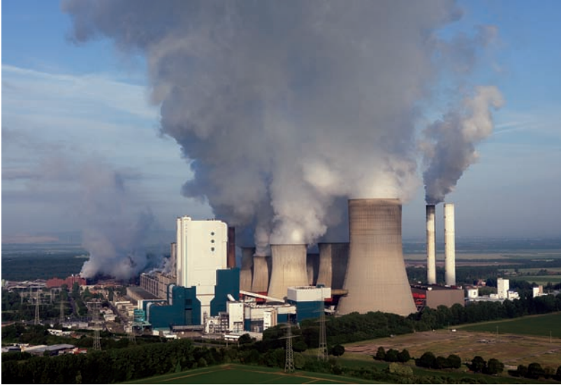
Fig. 2.9.3. The Niederaussem brown-coal power plant near Cologne, Germany. Coal-burning plants release carbon dioxide, fine particles, nitrogen oxide, and mercury, which can have a serious impact on public health. The coal ash produced by these plants contains contaminants such as arsenic, a known carcinogen.
