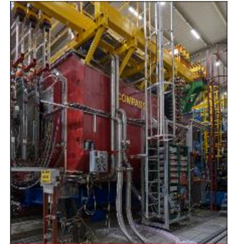
SM2-Dipole Compass-CERN 6953 MWh/y
