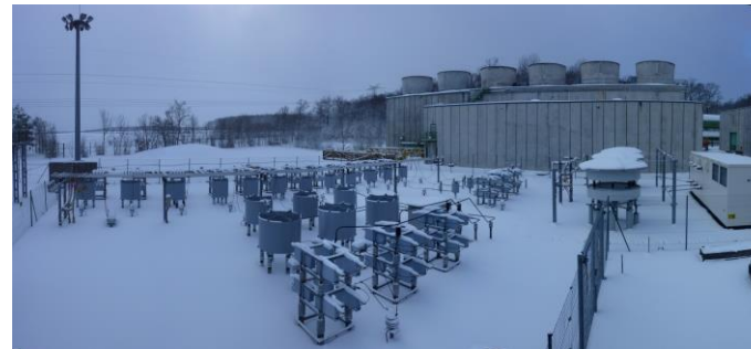
Static Var Compensator at CERN
