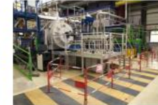
West Area test Facility
