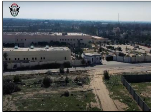
Figure 19.6 Exterior of Al-Maya DC b
