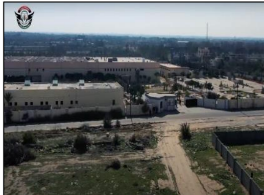
Figure 19.6 Exterior of Al-Maya DC b
