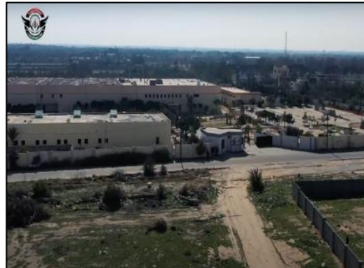
Figure 19.6 Exterior of Al-Maya DC b
