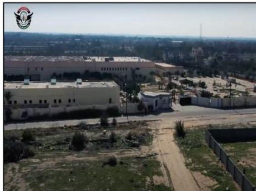
Figure 19.6 Exterior of Al-Maya DC b
