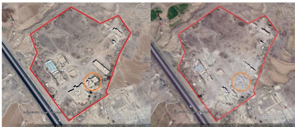
Satellite images of the Dhamar Community College compound (in red) before and after the airstrikes, of 30 January 2019 (left picture) and 21 October 2019 (right picture). Detention facility site circled in orange. (Source: Google Earth – Maxar Technologies)
