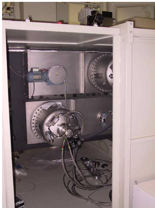
Fig.JRA1.2.8: Cryogenic pumping station with 20.000 l/s
