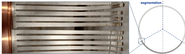
Figure 3: A sample photograph depicting the increased gap between two welded RF finger sheets.
