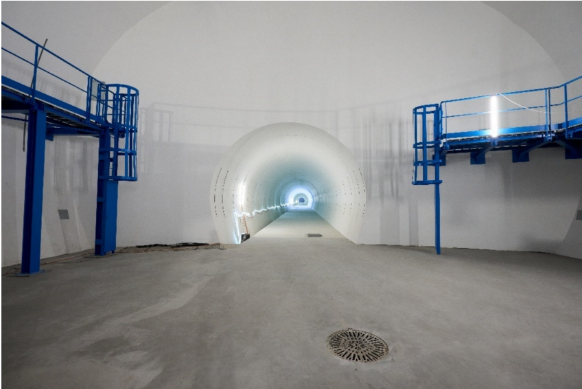
Fig. 20. HL-LHC underground cavern at Point 5.
